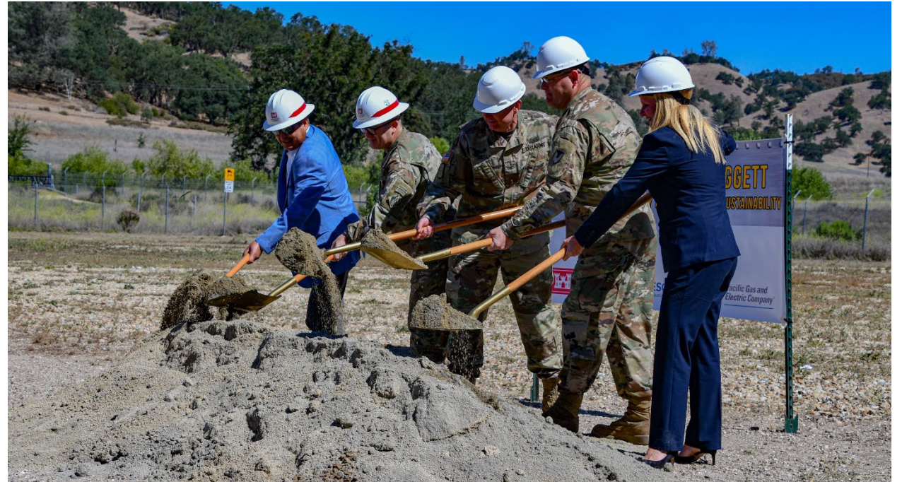
Fort Hunter Liggett breaks ground on its new microgrid project, May 2011
