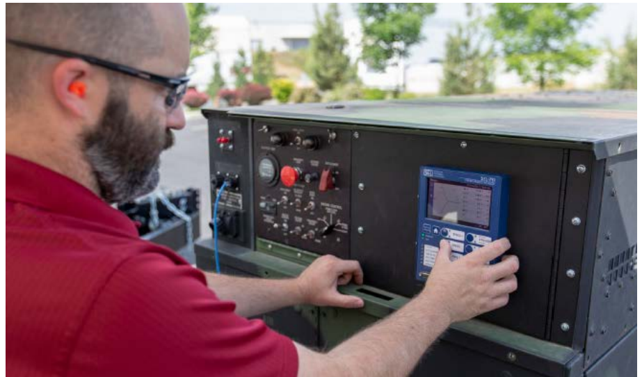
Figure 1: TQG After a Controls Upgrade (Photo Source: Author)
