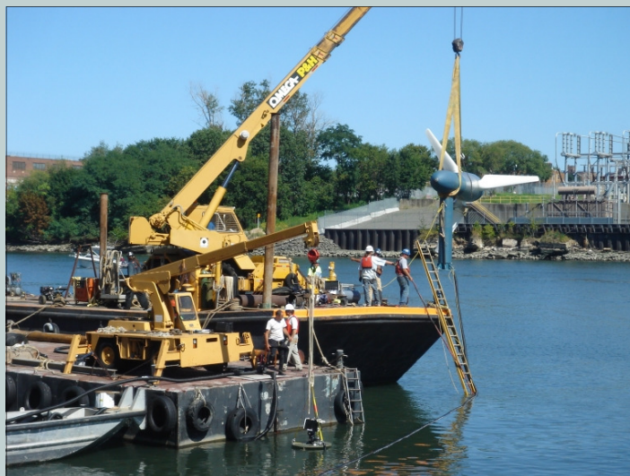
Verdant testing its tidal energy device in New York's East River. (Photo courtesy of Verdant Power/Released)
