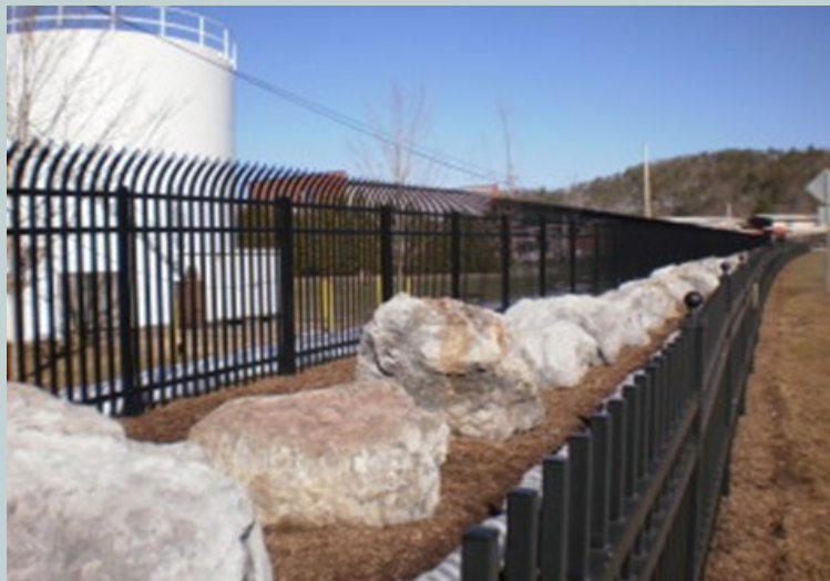
Example of Risk-Mitigation and Enhanced Outer-Perimeter Security. (Courtesy of William F. Booth, CPP/Released)
